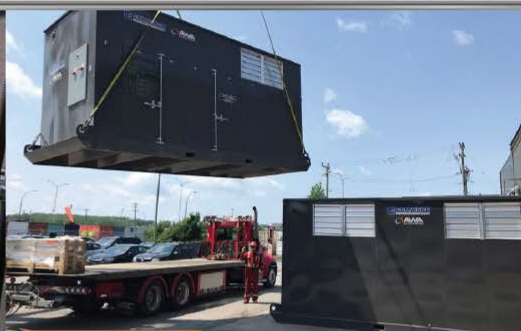
EASY HANDLING WITH LIFTING BRACKETS FOR CRANE
